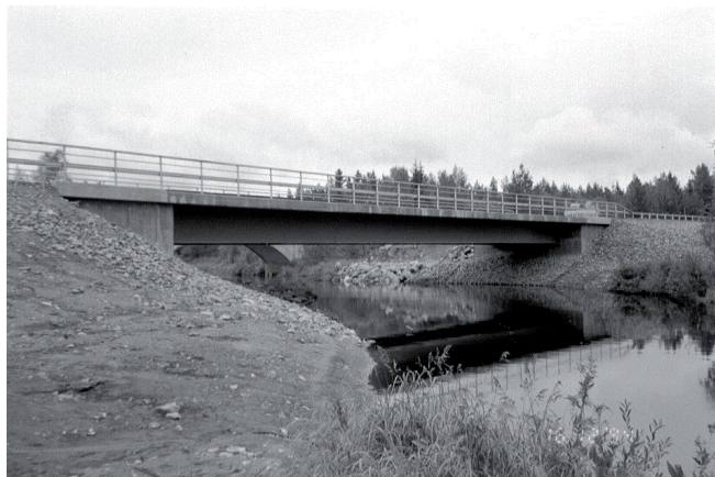
Fig. 3 Bridge over Fjällån after completion
