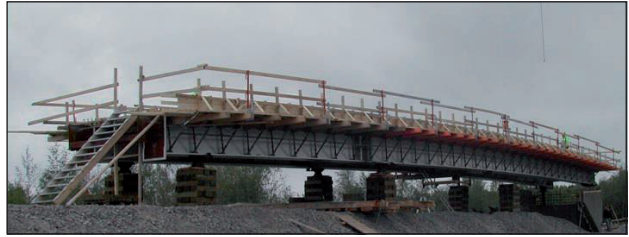
Fig. 6: The bridge superstructure before it was launched in place
