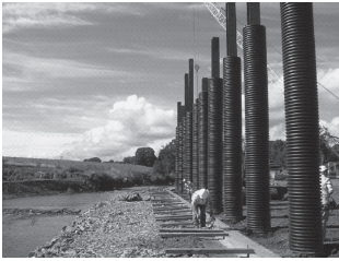
Fig. 3. H-piles in corrugated polythene pipe sleeves (Iles 2005, with permission from SCI)
