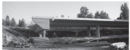
Fig. 6. Finnish FIAB with large diameter steel pipe piles during construction [picture by Anssi Laaksonen, Haavistonjoki Bridge Monitoring, Tampere University of Technology, with permission (Kerokoski 2006)]
