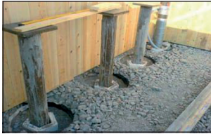
Fig. 5: Piles have been driven. The pile to the right was later used for monitoring. The picture shows the loose sand and styrofoam plates that were used to achieve a less stiff surrounding for the upper part of the piles
