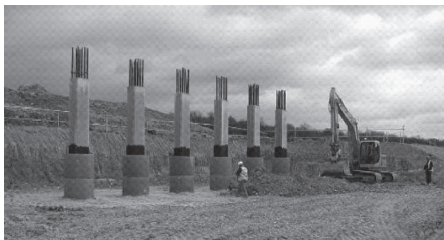
Fig. 4. Reinforced concrete piles inside concrete manhole rings (picture by David Price of Mott MacDonald Ltd., with permission)
