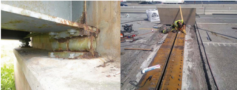
Figure 1 A leaking joint that has caused severe corrosion on the steel beams and bearings of the bridge in the left picture. Joints that need to be repaired or replaced cause much disturbance for traffic as shown in the right picture.
