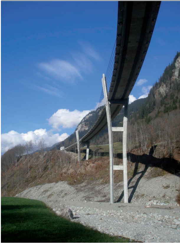
Figure 14 Sunniberg-Bridge in Switzerland (Picture by Dr. Ana M. Ruiz-Teran).
