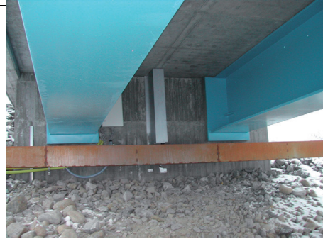
Fig. 16. Picture showing the northern abutment; the metal housing covers the displacement transducers; the reference beam in front is supported by two steel piles placed at sufficient distance from the bridge to avoid being affected by the bridge movements
